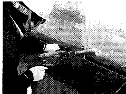
Picture 3: Shaving hole by drill
